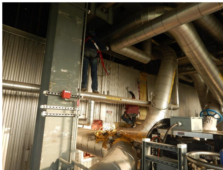
Penthouse dismantling started
