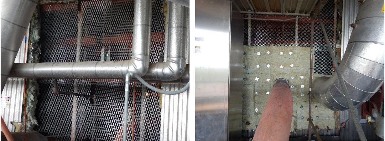
PH side framing on and starting insulation
