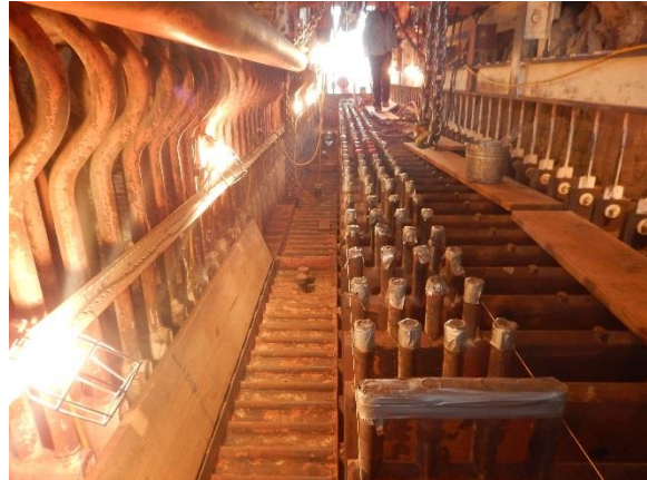
SH tubes prepped and ready for fit up
