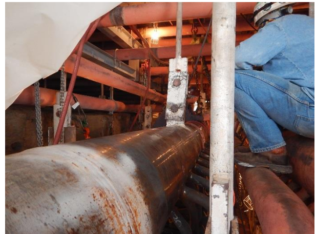
Header set and welding in progress
