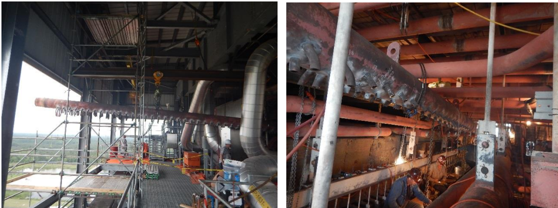
Old header cut out and hanging on monorail
