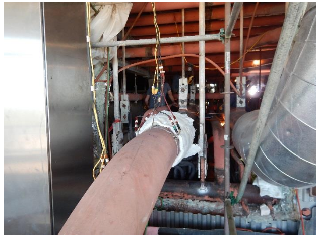
PWHT P91 joints on both sides
