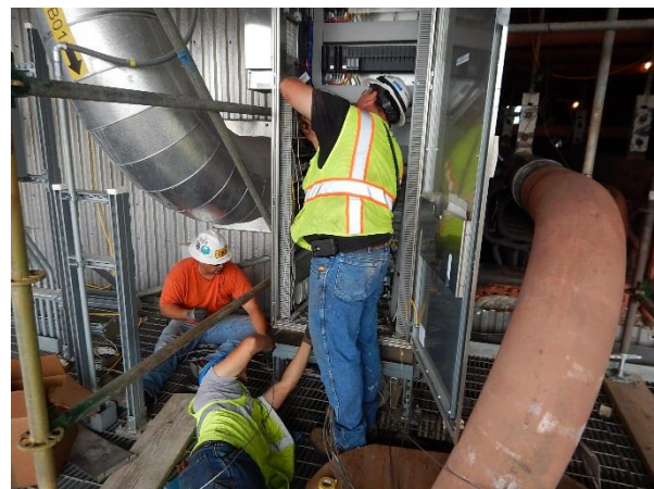
Installing Tertiary SH TC's
