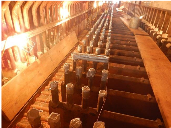
SH tubes prepped and ready for fit up
