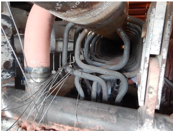
Installing Tertiary SH TC's
