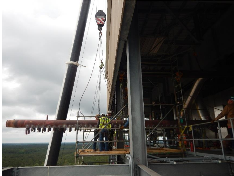
Tertiary header coming out from monorail to crane
