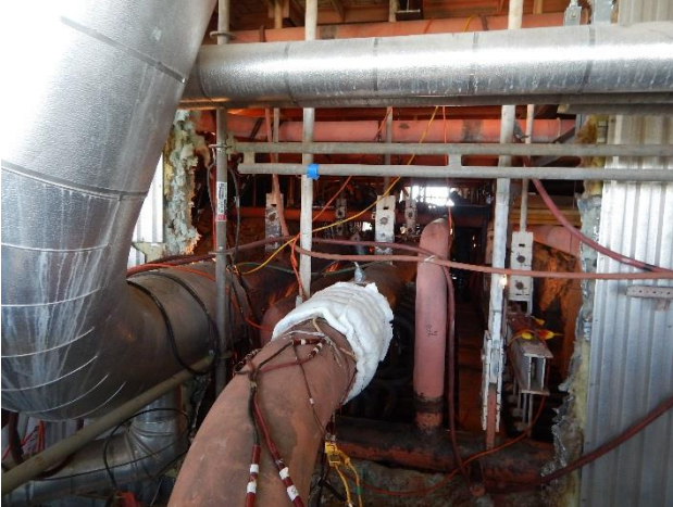
PWHT P91 joints on both sides
