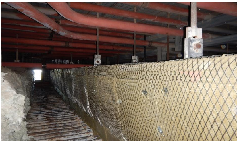
Tertiary and Primary SH reinsulated
