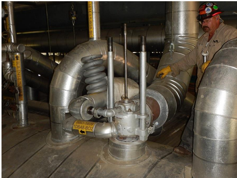
Installing hydro plugs on safety valves
