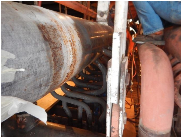
Header set and welding in progress
