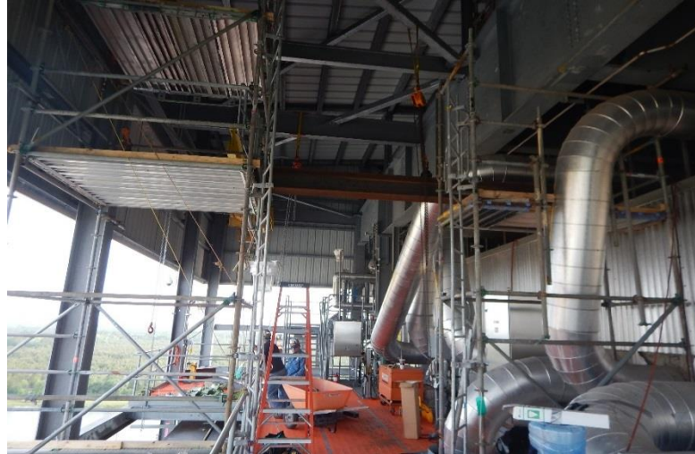
Monorail installation inside building
