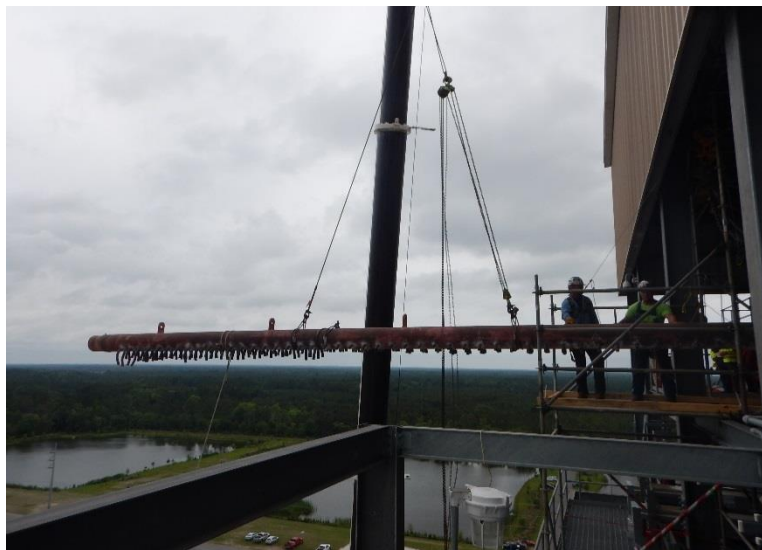
Tertiary header coming out from monorail to crane
